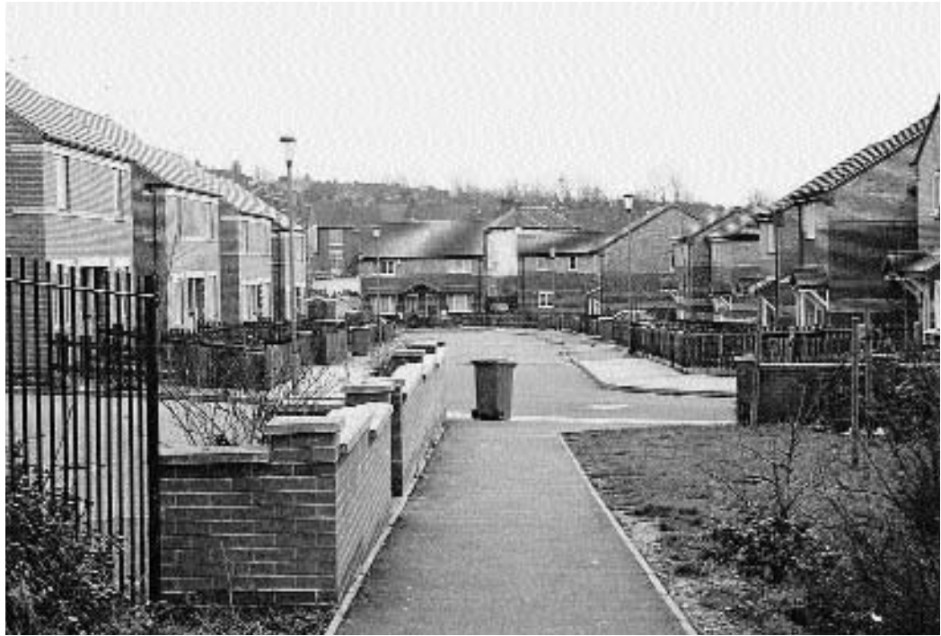
Figure 3.1 Radford. A return to a street architecture after demolition of 1960s deck access flats.
